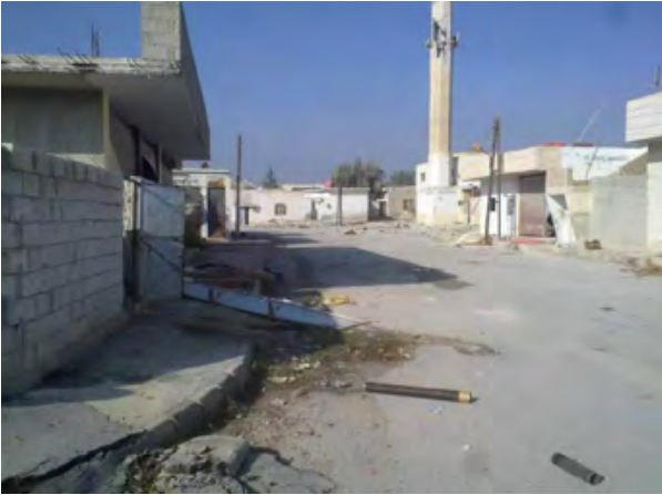
View of the street after an attack using explosive weapons, picture provided by an interviewee.
